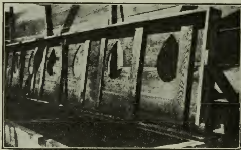
FIG. 77.—Latrine box, lid raised for treatment by oil and lamp black. This mixture is strained immediately before use through a sieve made of two layers of wire mosquito net tacked to a square wooden frame 8 inches square and 1 inch deep.
